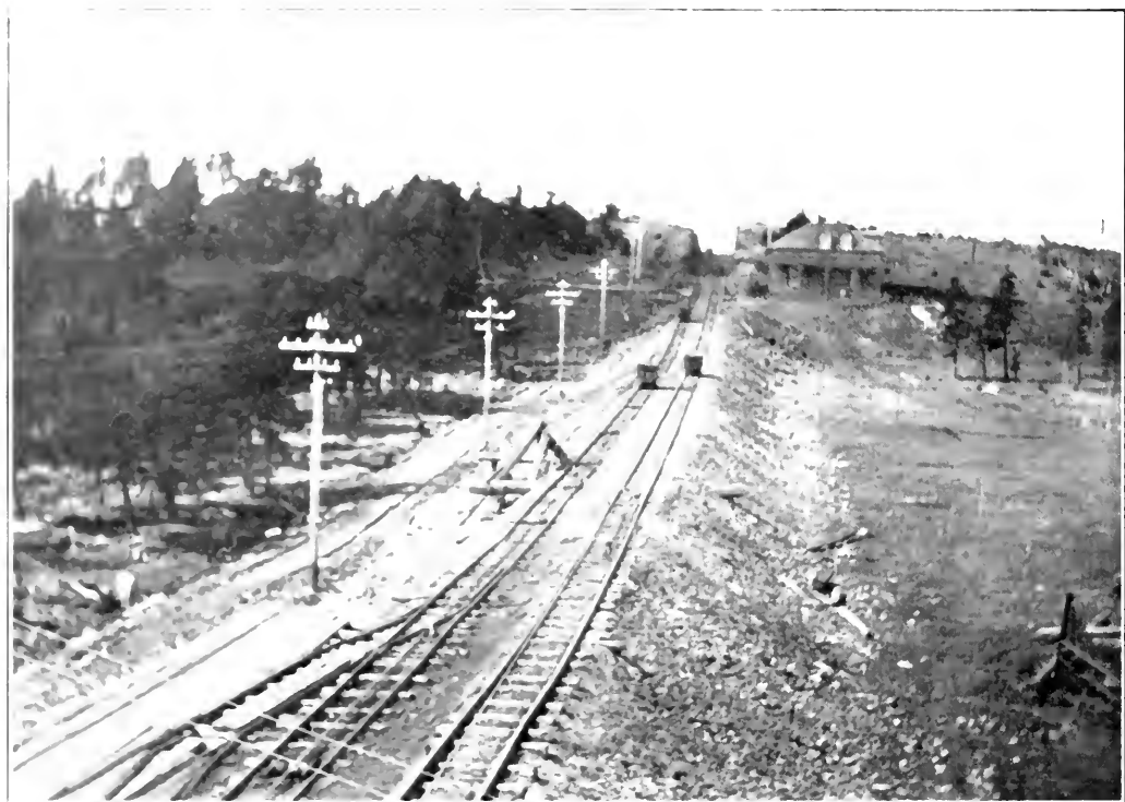
Cable-operated Tramway from Pier to Mine, at Wabana Iron Mines.
